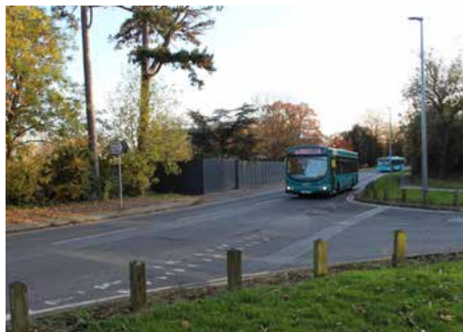
View south along Sherwood Drive with former Fire Station behind temporary fencing
