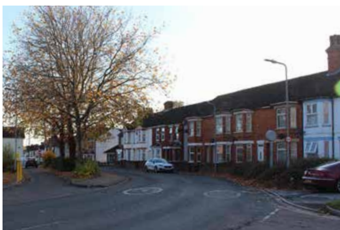
Typical Victorian terrace alongside town centre
